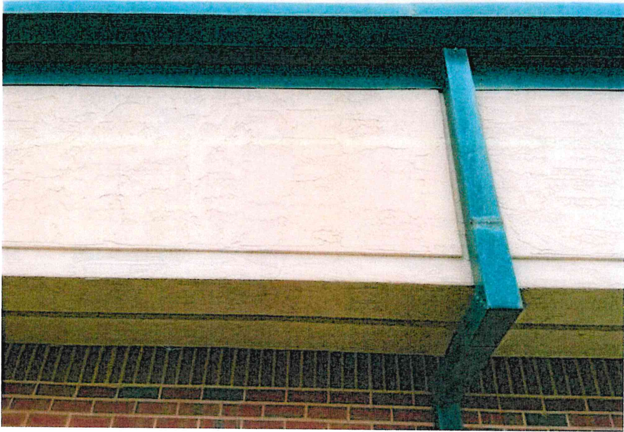
EIFS Section on building envelope
