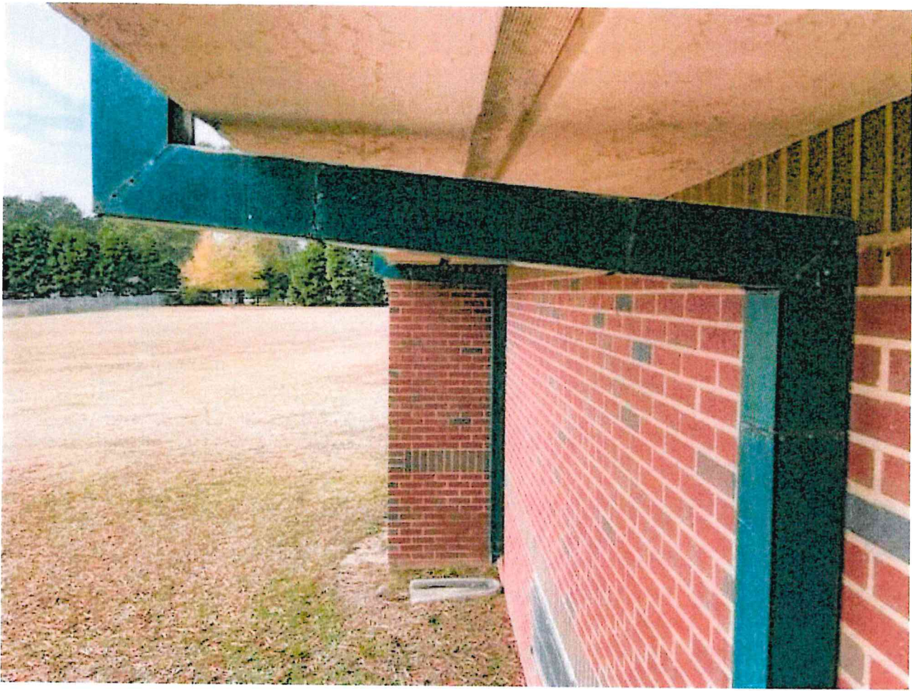
EIFS attached with proper spacing above gutter downspout
